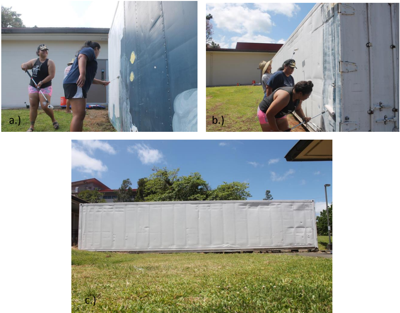
Figure 6. a and b) Leilua and Natasha applying 3 coats of primer. c) View of the container after applying 3 coatings of white primer on the surface (2017).
